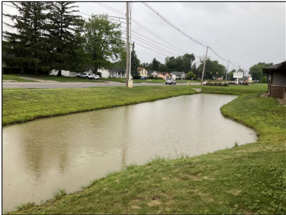
Photo 26: View of manmade pond adjacent to Karl Rd., facing north.
