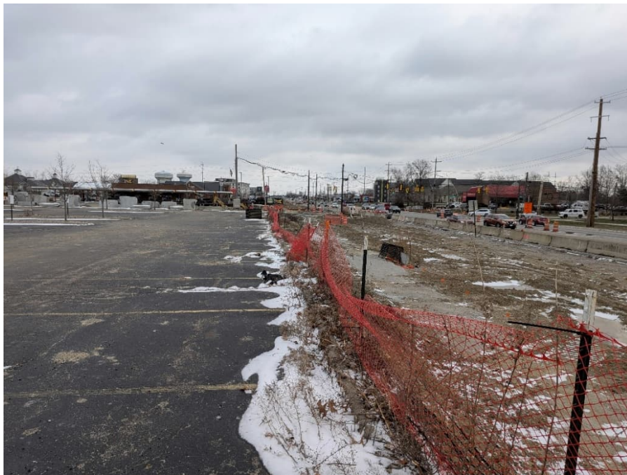
Photo 6: View towards Project from FRA1107506, facing east.
