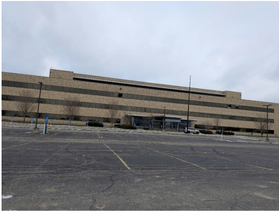
Photo 5: Oblique view, industrial building, FRA1107506, facing north.
