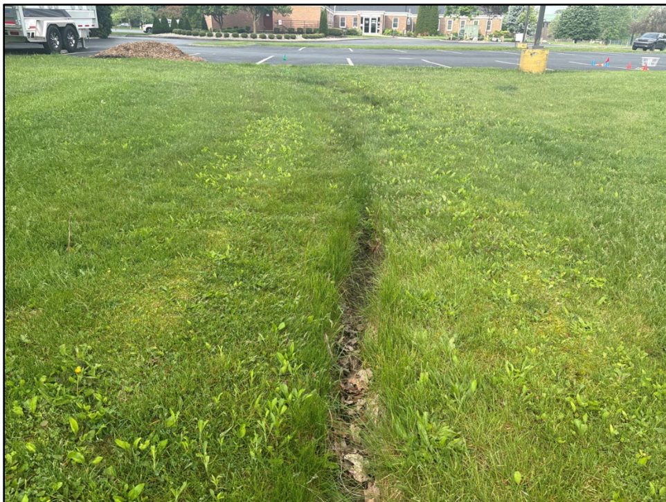
Photo 8: View of ditch (D)1, facing southwest.
